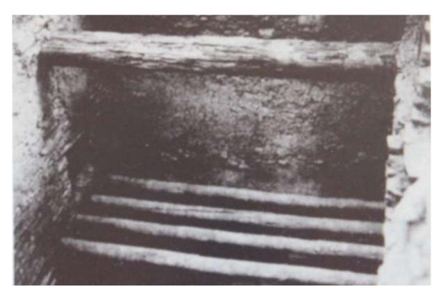
Figure 7.4.3-1: A room in Chaco with built-in log rails spanning from side to side. The logs were inserted in the stone walls at the time of original building construction indicating that whatever was to be placed on them was of very high priority (photograph from Lekson 2015).
